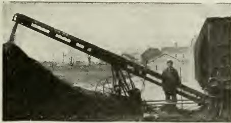
Fig. 1.—Unloading from coal car to storage pile with a Scoop Conveyor.
